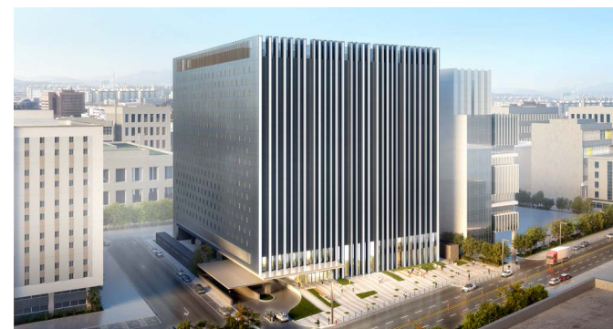
Aerial view of Gasan Data Center
